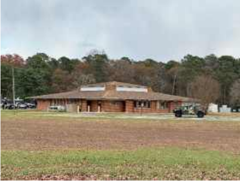
STATE OF DE STOCKLEY CAMPUS, COTTAGE C-1 9,000 SF EXISTING BUILDING
